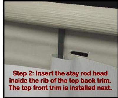
Step 2: Insert the stay rod head inside the rib of the top back trim. The top front trim is installed next.
