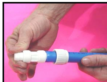
▲ Step 2- Insert fitting into tubing until it rests against the fitting threads.
